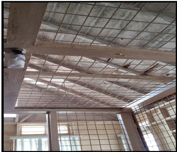
Moruga Magistrate Court, Roofing
